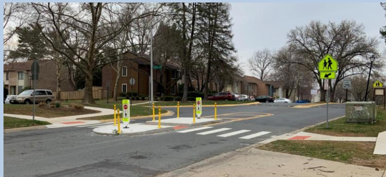
An Island Was Installed North of Whetstone Elementary School
