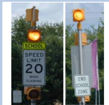
Rear-Facing Beacon Installation
