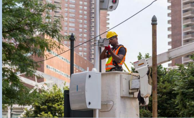
Installation of A SSC
