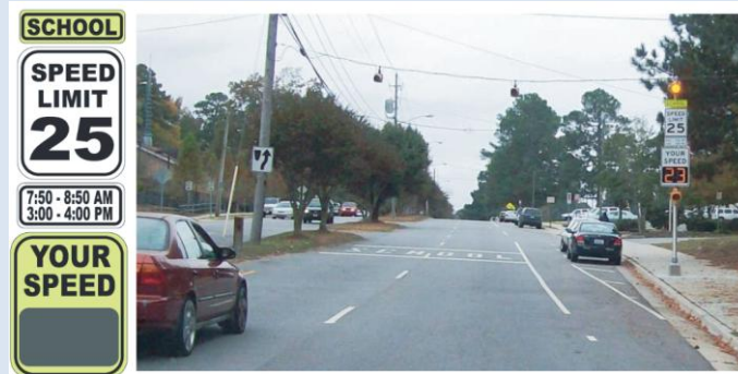
"School Speed Limit" Sign Assembly Incorporating "Your Speed" Sign
