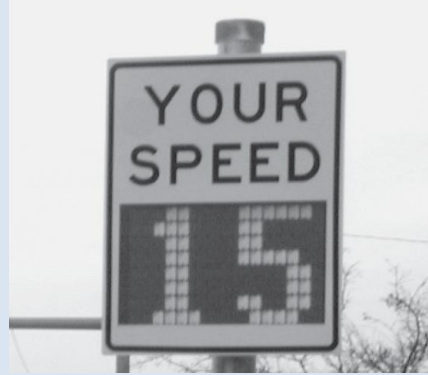
Example of Permanently Installed Self-contained DSDS Units
